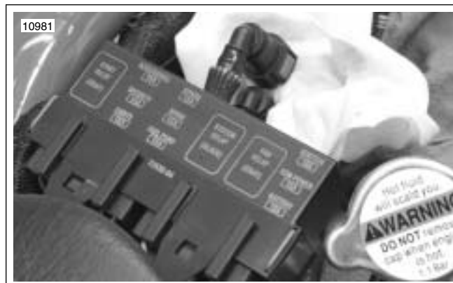
Figure 8-87. Fuse Block Location
